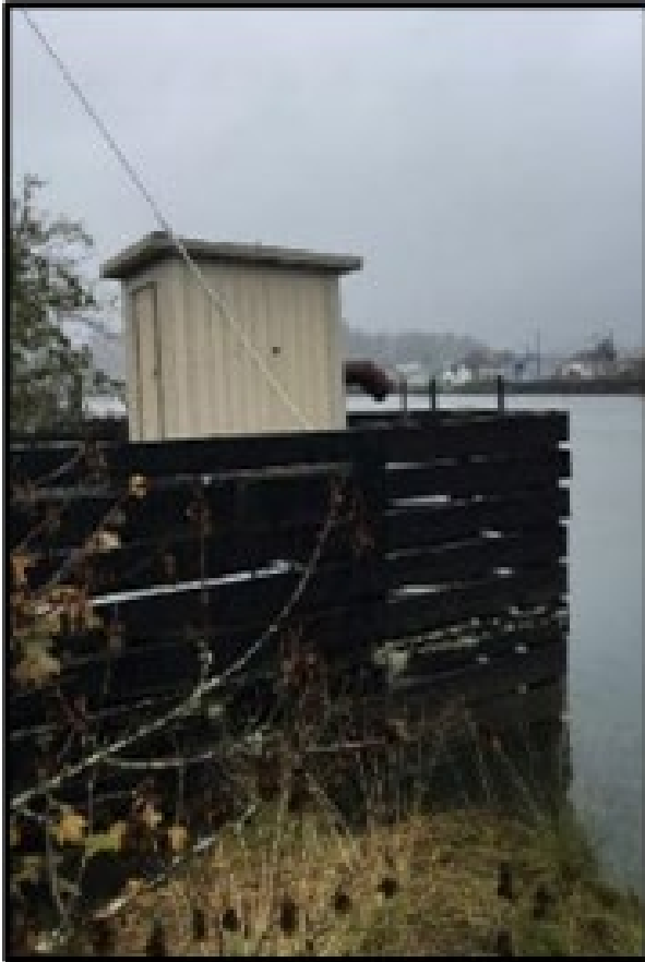
Pic 7 -- 10th St. Pump Station
