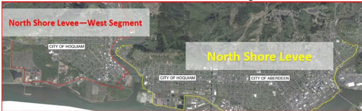
Pic 6 -- North Shore Levee with West Segment
