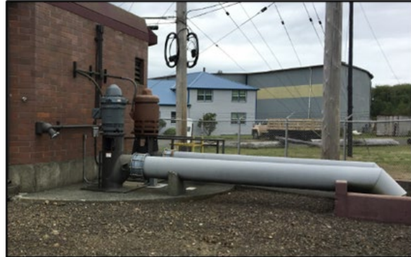
Pic 8 -- Queen Ave. Pump Station
